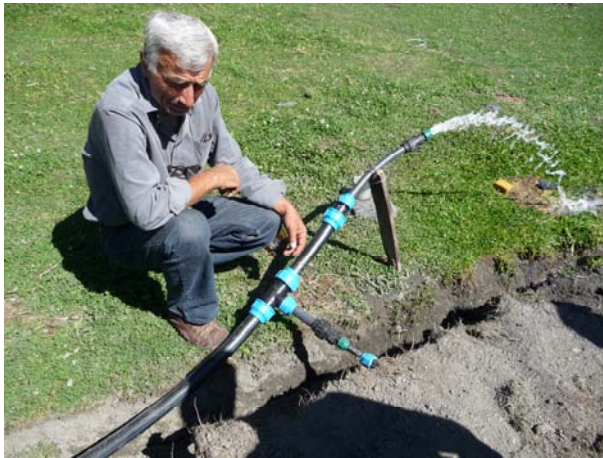
Photo 4: Testing water pressure in Dano
